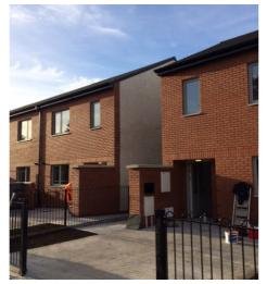
The external façade of the houses is built with an external leaf either brick or plastered blockwork tied back to the LGSF frame with abbey
