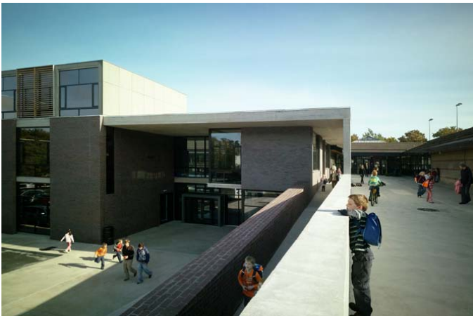
Image 1 - Showing New & Existing School
