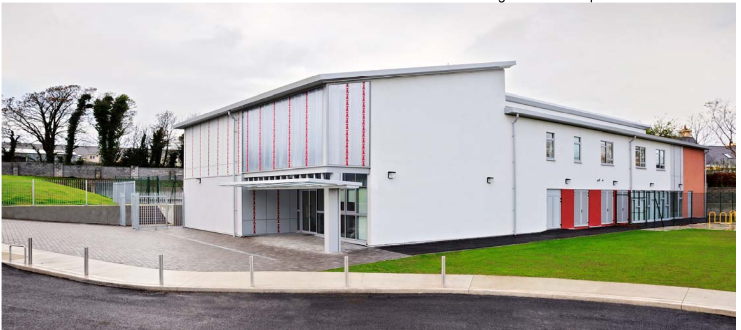
Image 1- View of West Elevation
