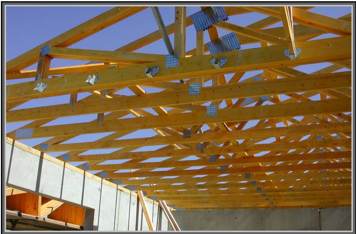
Image 5 - Precast wall system with prefabricated roof truss
