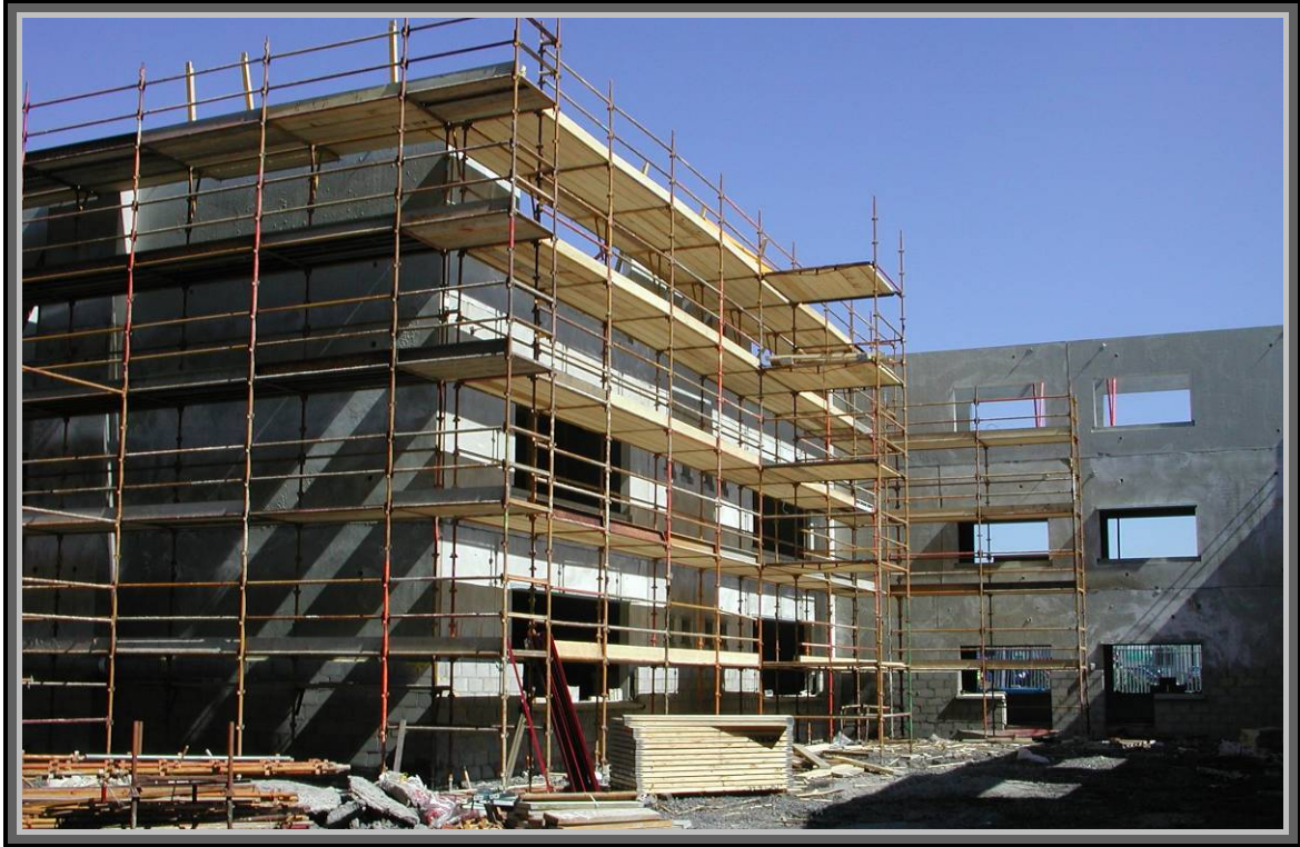
Image 4 - Precast wall system erected to three storeys
