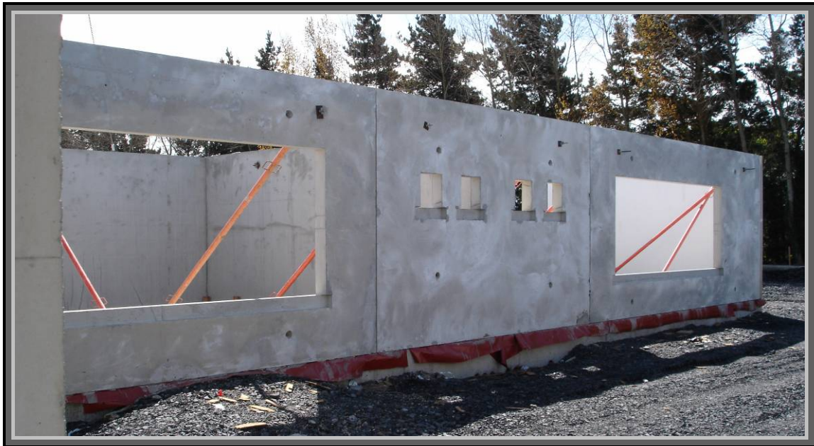
Image 2 - Precast wall system erected at ground floor level
