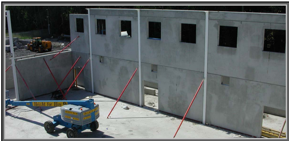
Image 3 - Precast wall system erected to two storeys
